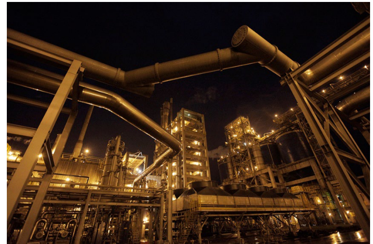
World largest carbon black plant Tianjin, China
